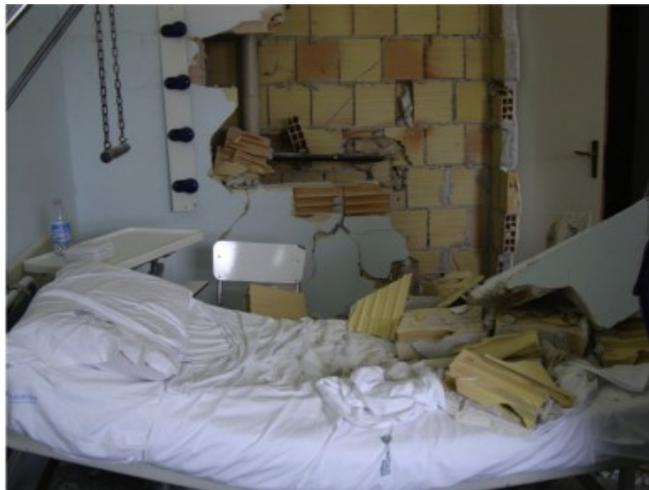
**Figure 1.2 - Damages recorded in San Salvatore hospital brick partitions, after the L'Aquila earthquake in 2009**
