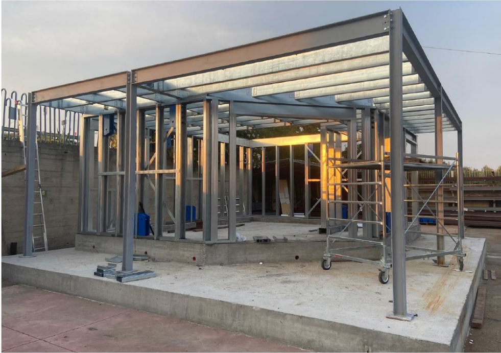
i) Complete first storey structure
