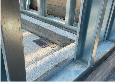
d) Gravity frame track-to-stud connection
