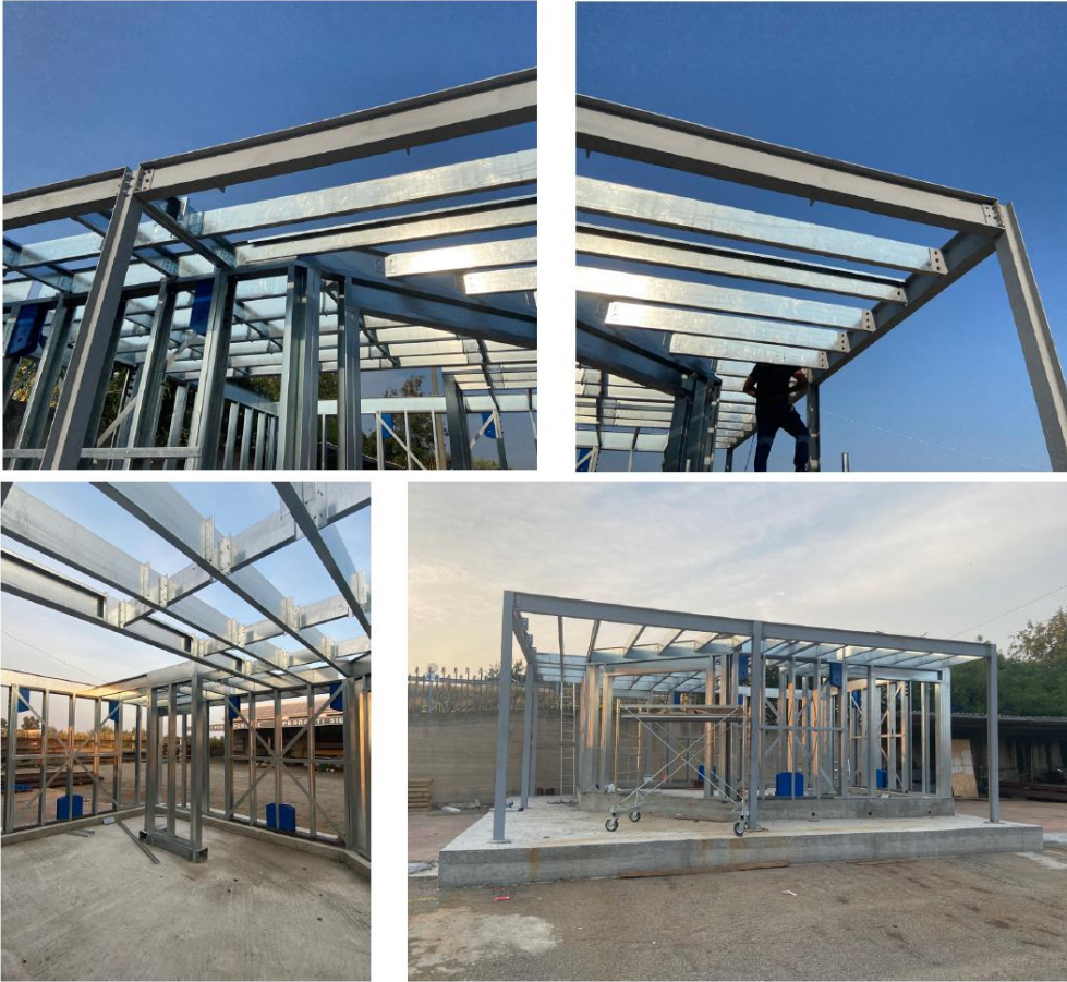
k) Different views of steel structures
