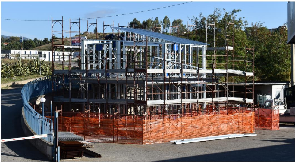
l) Complete structure
