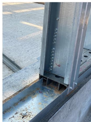
b) LFRS and gravity frame connection
