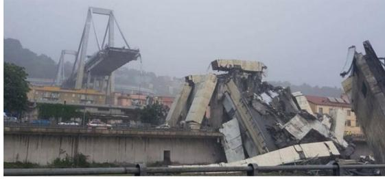
**Figure 2.1.** The collapse of the “Polcevera” viaduct
