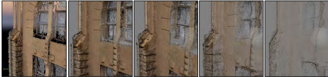
Figure 3.20: Detail of the column and window in segment three: Pix4D (left), then PhotoScan from high to lowest accuracy (right)
