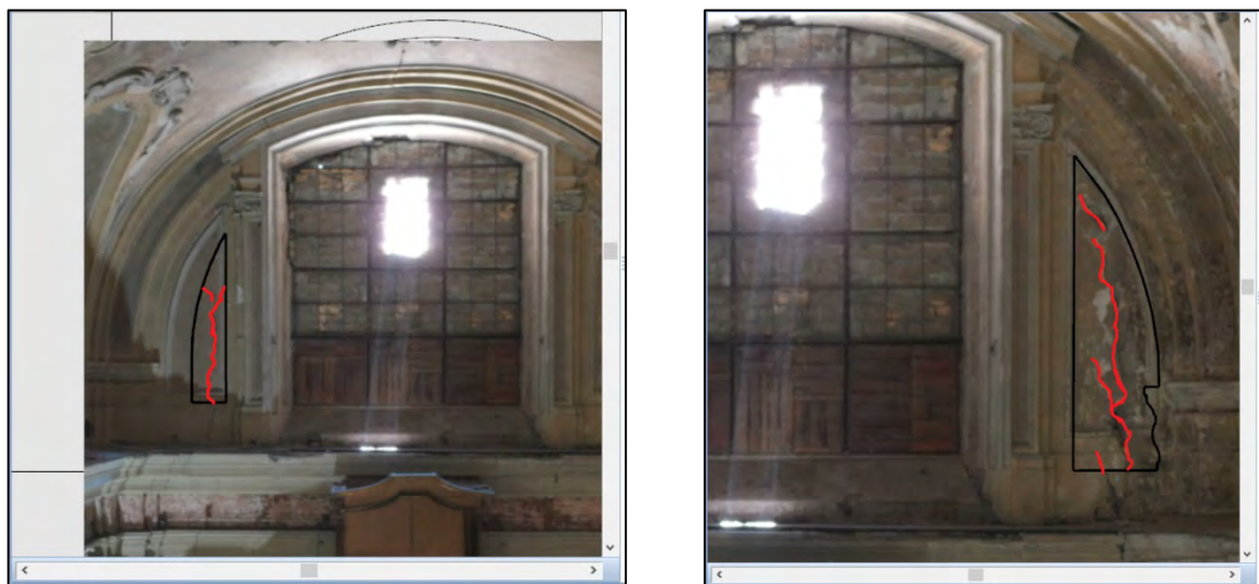
Figure 6.24: Crack modelling
