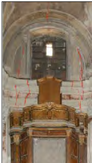
Figure 6.8: Cracks on the main façade of the San Pietro in Vinculis church
