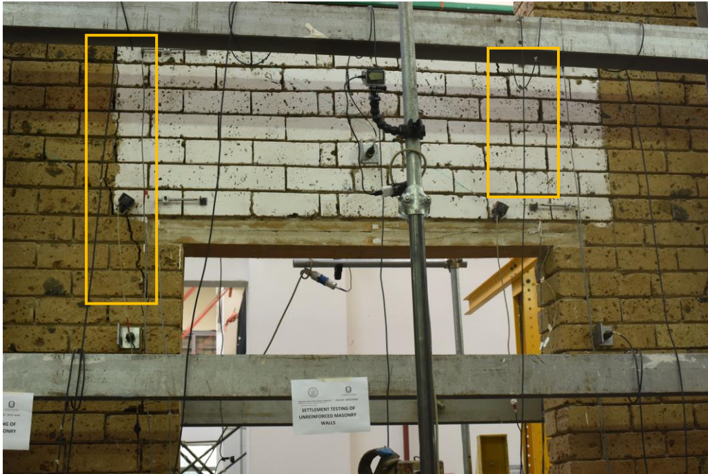
Figure 45. Crack pattern at 35mm of settlement applied to deteriorated URM, frontal side
