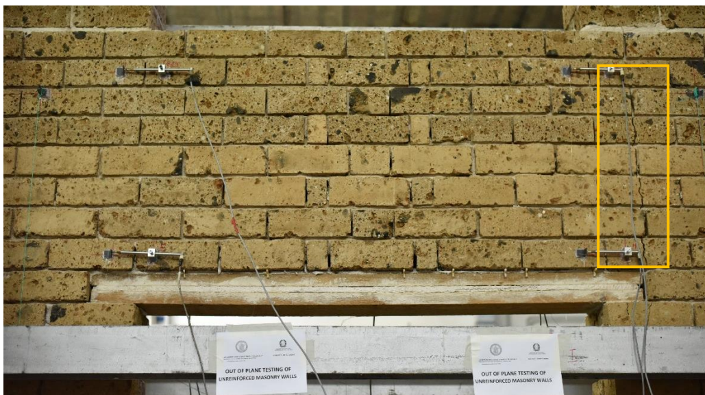
Figure 63. Crack pattern for spandrel, deteriorated URM, back side
