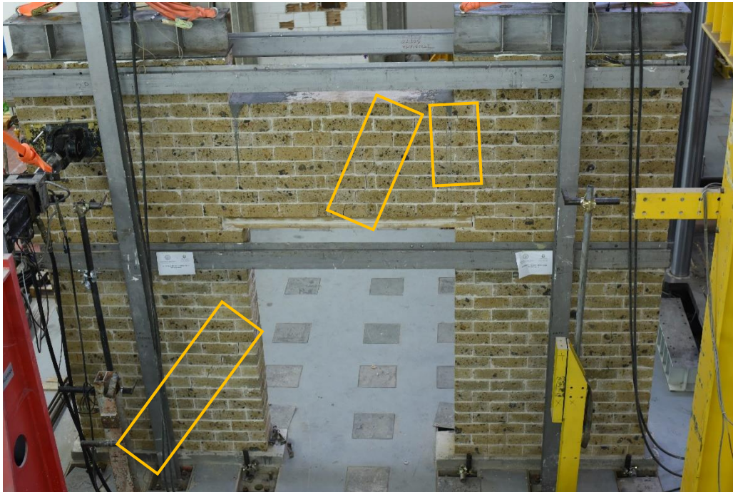
Figure 54. Crack pattern for intact URM, frontal side
