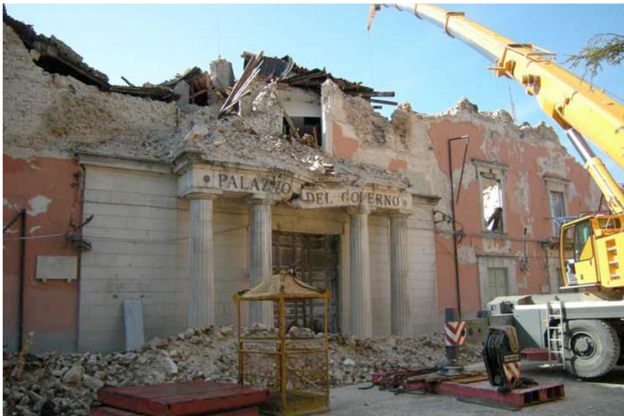
Figure 6. Global collapse of the L'Aquila's Prefecture. Photo retrieved from Augenti and Parisi, 2010.
