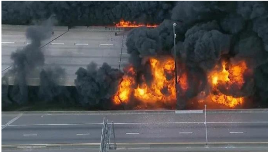
Figure 1.2. Massive fire causing collapse of an overpass on Interstate 85 in Atlanta, US, 2017 [5]
