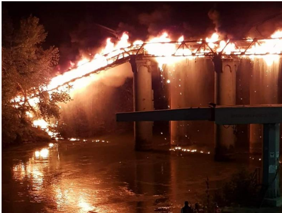
Figure 1.1. Fire event on “Ponte di Ferro” in Rome, Italy, 2021 [4]
