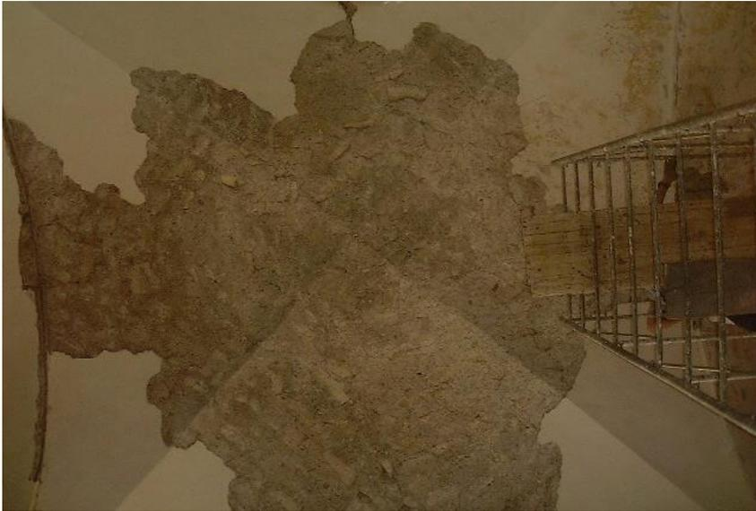
Figure 4.14. Cross vault of construction 0 after the 1980 Irpinia Earthquake: herringbone arrangement.
