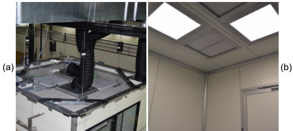
Figure 3.5: View of the assembled ceiling system: (a) from the top and (b) from the inside the cleanroom.
