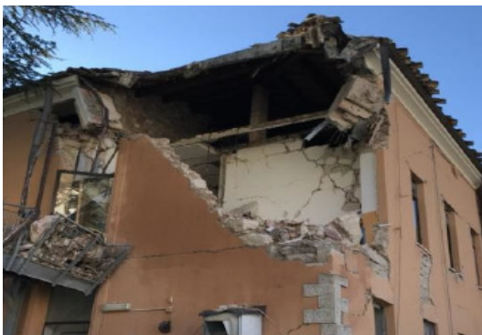
Figure 1 – Corner failure
