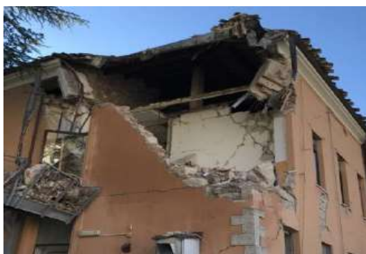
Figure 1 – Corner failure
